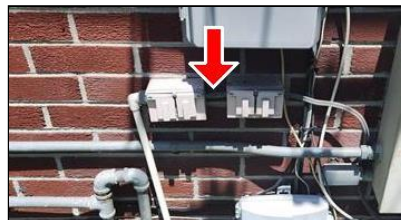
6.5 Item 3(Picture) Example/ Sample- Rear of Home
