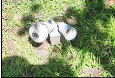
6.7 Item 1(Picture) Example/ Sample- Front of Home
