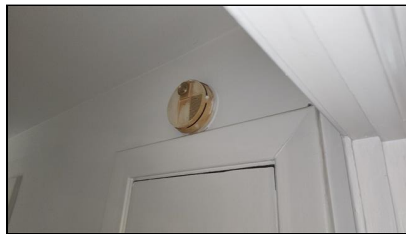
6.11 Item 1(Picture) Example/ Sample- First level Hallway
