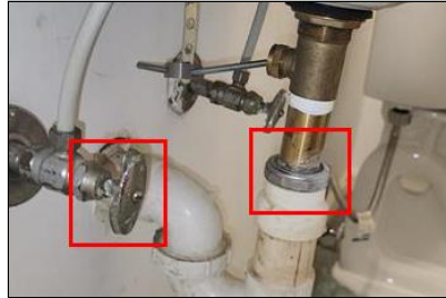
5.4 Item 2(Picture) Example/ Sample- Second level Bathroom
