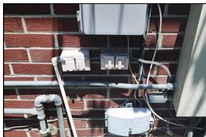
6.9 Item 2(Picture) Example/ Sample- Rear of Home
