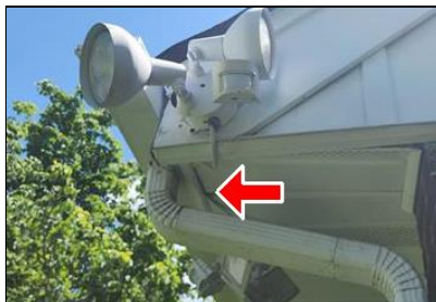
6.5 Item 2(Picture) Example/ Sample- Front of Home
