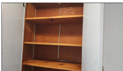
6.5 Item 5(Picture) Example/ Sample- Kitchen
