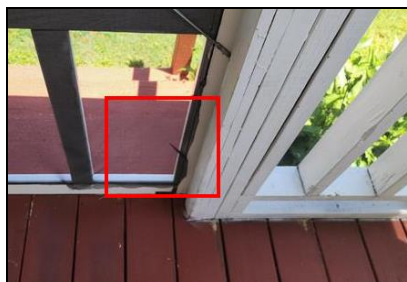
3.6 Item 1(Picture) Example/ Sample- Enclosed Deck
