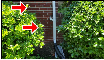
2.0 Item 6(Picture) Example/ Sample- Front of home- cracking
