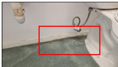
3.0 Item 10(Picture) Example/ Sample- Second level Hall Bathroom
