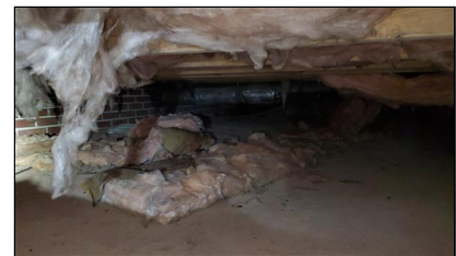
8.1 Item 3(Picture) Example/ Sample- addition crawlspace
