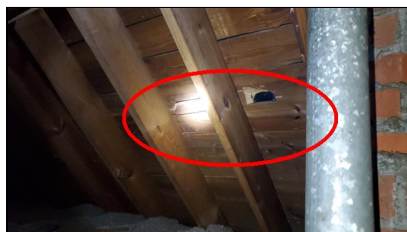
4.2 Item 1(Picture) Example/ Sample- front of home – near the chimney
