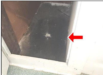
3.1 Item 3(Picture) Example/ Sample- Second level Bathroom
