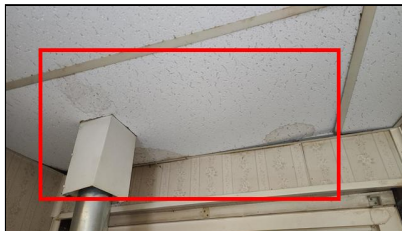
3.0 Item 5(Picture) Example/ Sample- Laundry Room
