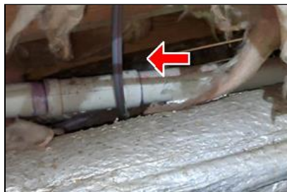
5.4 Item 12(Picture) Example/ Sample- addition crawlspace
