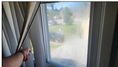
3.6 Item 7(Picture) Example/ Sample- Second level Left Bedroom
