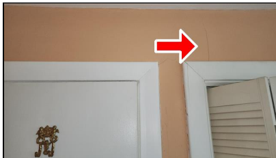
3.0 Item 16(Picture) Example/ Sample- Rear Right Bedroom
