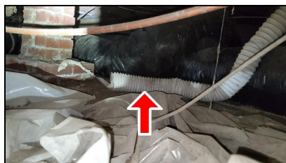
8.4 Item 1(Picture) Example/ Sample- located near the front of home
