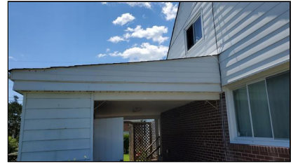
1.0 Item 12(Picture) Example/ Sample- carport area
