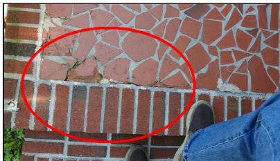
2.2 Item 1(Picture) Example/ Sample- front of home – porch
