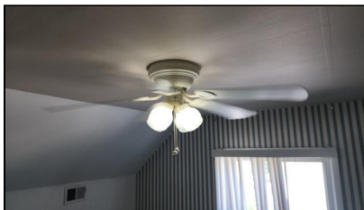
6.8 Item 1(Picture) Example/ Sample- Second level Left Bedroom
