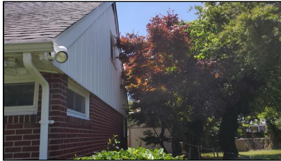
2.2 Item 3(Picture) Example/ Sample- Right side of home-
