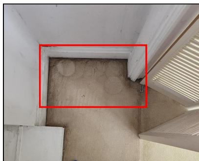
3.0 Item 7(Picture) Example/ Sample- Rear Left Bedroom Closet
