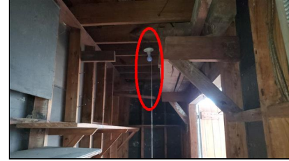
6.7 Item 3(Picture) Example/ Sample- shed at car port area
