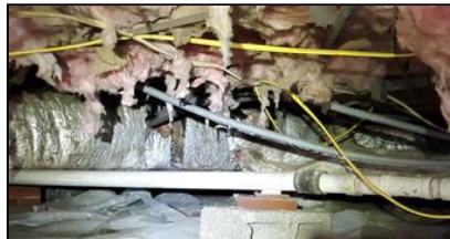
8.1 Item 4(Picture) Example/ Sample- crawlspace
