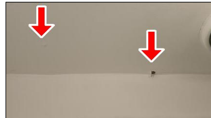
3.0 Item 18(Picture) Example/ Sample- Second level Hall Bathroom
