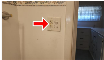
6.4 Item 2(Picture) Example/ Sample- Second level Bathroom
