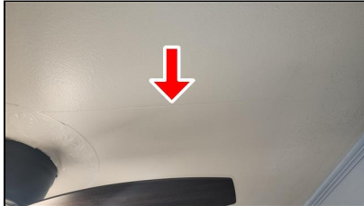
3.0 Item 13(Picture) Example/ Sample- Kitchen
