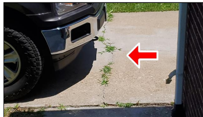
2.2 Item 2(Picture) Example/ Sample- driveway
