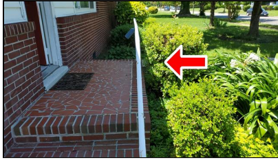
2.1 Item 8(Picture) Example/ Sample- Front of home-
