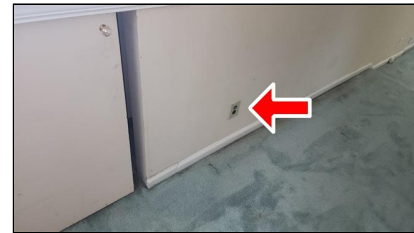
6.4 Item 3(Picture) Example/ Sample- Second level Den
