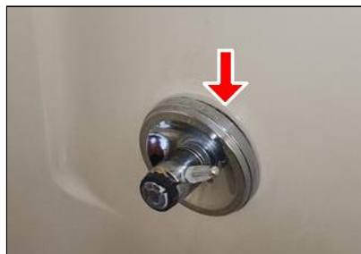
3.0 Item 20(Picture) Example/ Sample- Laundry Room Shower
