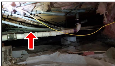
5.4 Item 13(Picture) Example/ Sample- crawlspace
