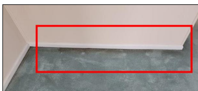
3.1 Item 2(Picture) Example/ Sample- Second level Right Bedroom
